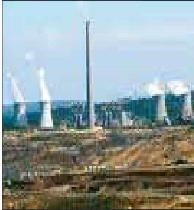
Central térmica de As Pontes
